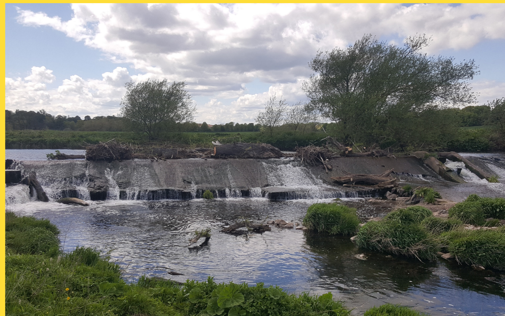
Knowes Weir with debris and no working fishway, River Tyne, Scotland, UK © Forth Rivers Trust
